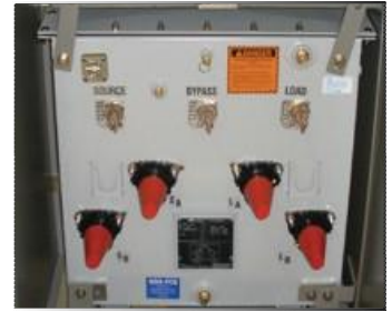
Single-phase bypass module
