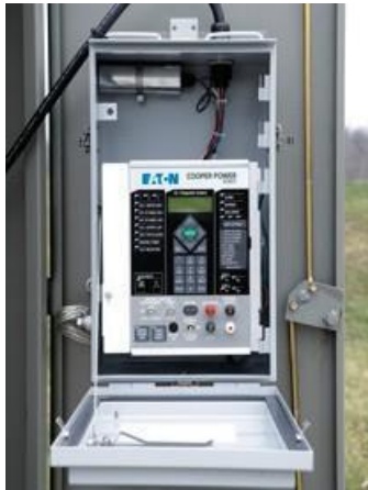
Door-mounted CL-7 single-phase control
