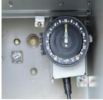
Standard gauges and provisions for single-phase pad-mounted regulator
